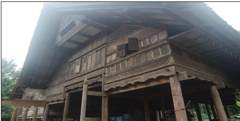
Figure 3. Aceh House Side View (Source: Data Analysis, 2023)
