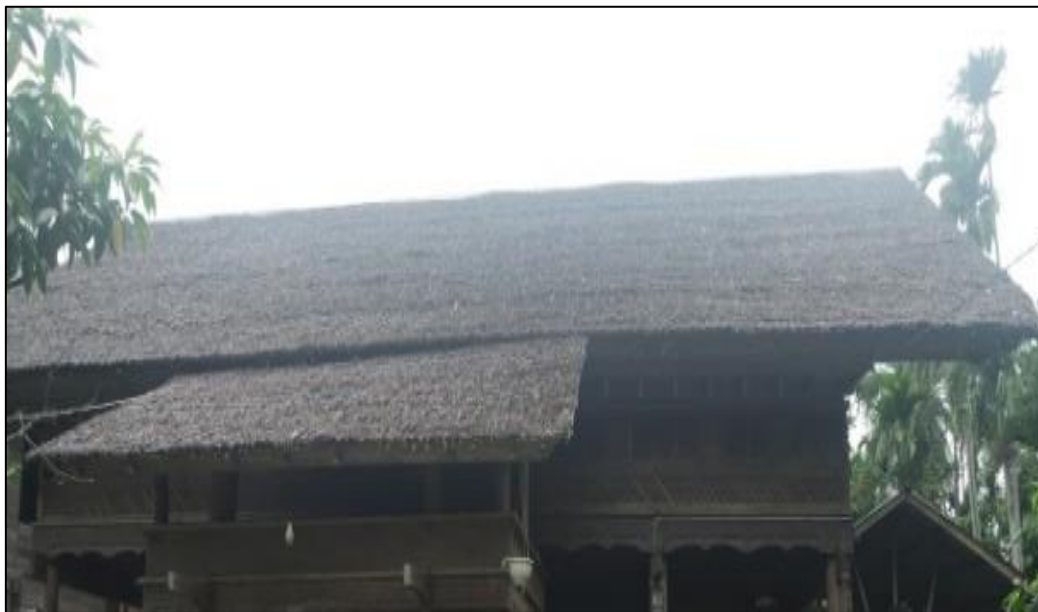
Figure 10. Roof (Source: Data Analysis, 2023)
