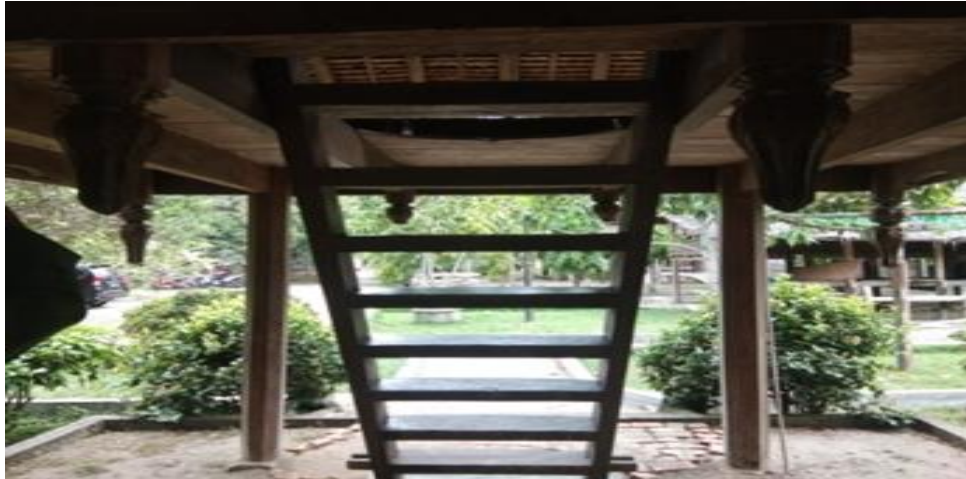
Figure 6. Stair (Source: Data Analysis, 2023)
